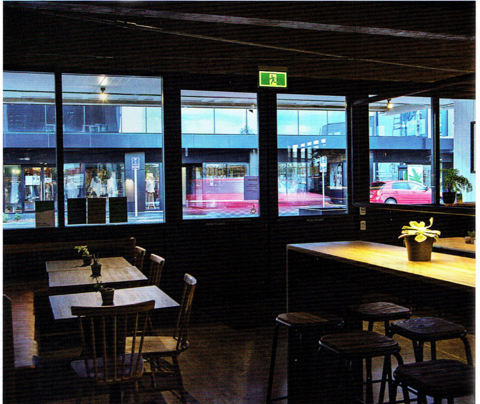
Hybrid PL signs, charged by their own dedicated light source, are reportedly appropriate for areas with poor ambient lighting.
