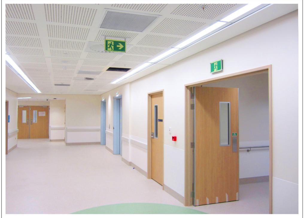
*Ecoglo International's HYU 'hybrid' exit signs are equipped with their own LED light source, which ensures the photoluminescent material in each exit sign is always fully charged even if ambient lighting is poor.*
