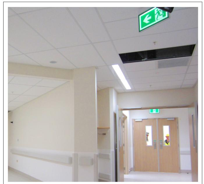
"Power consumption represents only about 5% of the overall running costs of an illuminated sign," Mark says. "A passive PL sign has zero electrical costs, while a hybrid 2.25W PL sign with LED lights might have an annual energy cost of about \$5.50; by contrast, a typical 4.5W illuminated sign can cost more than \$11 to run per annum. However, the really serious cost burdens lie in
